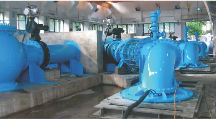
In this installation, the low suction sets had to fulfil very strict operating requirements and their design had to be suitable for the existing electrical installation. Three duty points with a minimum hydraulic efficiency had to be guaranteed and other technical requirements were mandatory.
