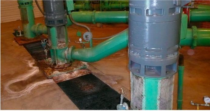
Because of the limited space (height and length) it was not possible to provide the new flow requirement of 12,000 GPM (2,725 m<sup>3</sup>/h) with traditional vertical turbine pumps. INDAR inverted submersible pumps and motors were selected to fulfill the requirement.
