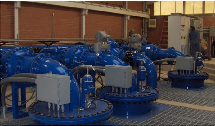
This picture shows the three, 300 HP (225kW) submersible pumps in line.
