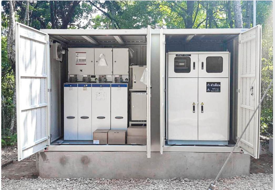
The objective of this project is to guarantee the **remote control and automation** of a ring main network used for distribution of power to the **King Palace** project, located in **Sakon Nakhon, Thailand**. Protection and control of this 24 kV urban secondary network is accomplished through four SF6 Gas Insulated RMU.
