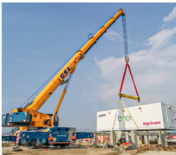
Unloading of the pre-fabricated hut with a crane
