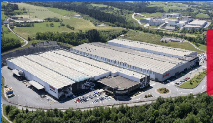
Electric machines manufacturing plant Beasain (Gipuzkoa)
