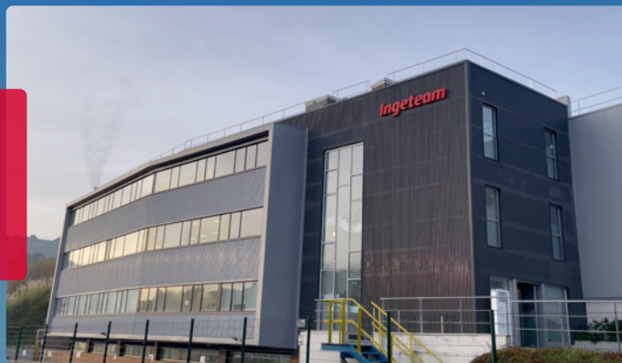
Power converters manufacturing plant Ortuella (Bizkaia)
