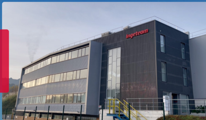
Ortuella (Bizkaia) Power converters manufacturing plant
