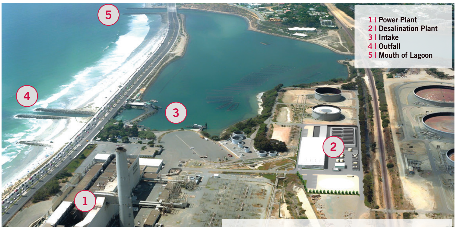
Figure 1. The Claude “Bud” Lewis Carlsbad Desalination Plant. The Largest, most technologically advanced and energy-efficient seawater desalination plant in the USA (Reverse Osmosis)
