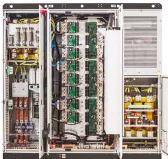
3.6 MW DFIG Power Converter
