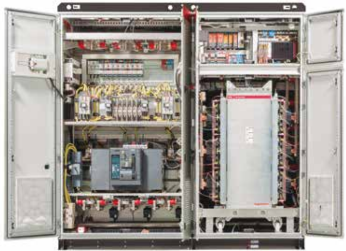
3.7 MW FC Power Converter
