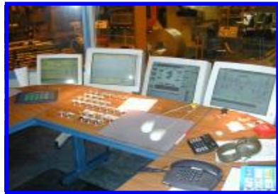
Main Control Pulpit
