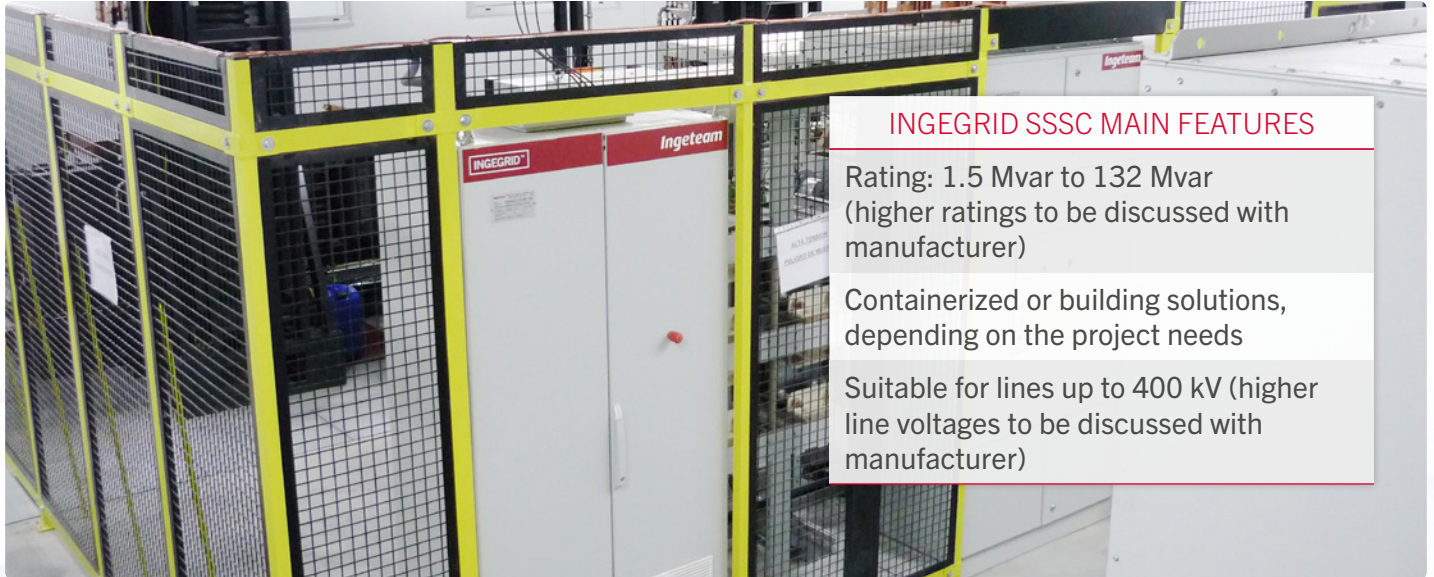
INGEGRID SSSC in Torres de Segre substation (220 kV) in Spain
