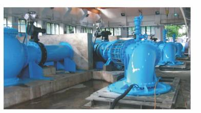
In this installation, the low suction sets had to fulfil very strict operating requirements and their design had to be suitable for the existing electrical installation. Three duty points with a minimum hydraulic efficiency had to be guaranteed and other technical requirements were mandatory.
