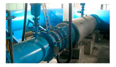
The space required by horizontal pumping sets was less than the vertical type sets needed. And the old motors generated a lot of noise and high heat. Indar submersible sets in horizontal configuration between pipes solved all these inconveniences.
