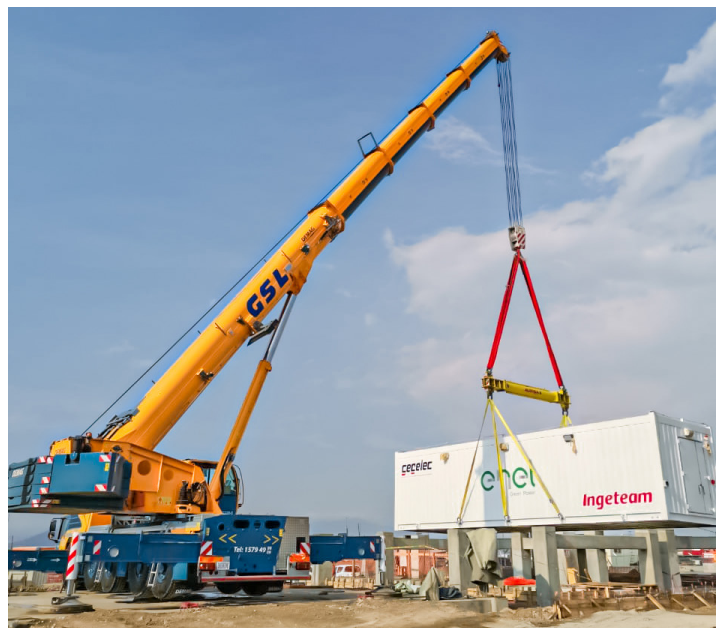
Unloading of the pre-fabricated hut with a crane
