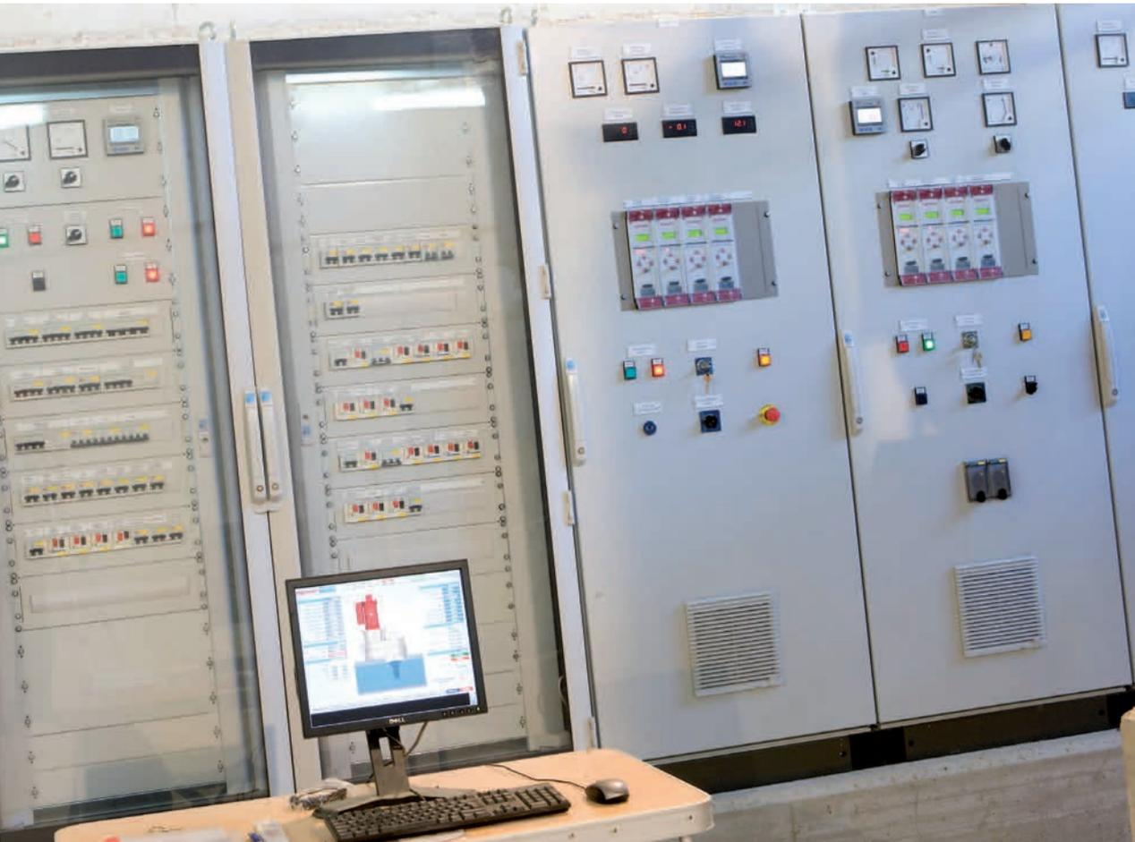
The Substation and any other device capable of being remotely controlled can be integrated into the Remote Control system, being compatible with many different protocols and media (ADSL, RDSI, GSM, GPRS, In-ternet, fibre optics, radio, micro-wave, satellite).
