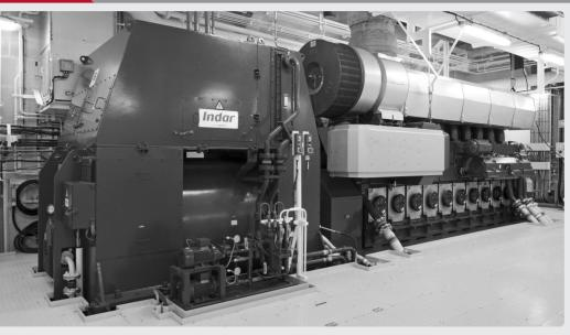
The basic concept of our INDAR SGI generator series (driven by Internal Combustion Engines where burning fuels are fossil fuel, biofuel, gas...) is its adaptability to the standards of each manufacturer. There are two variants: one for marine applications (SGIm Series) and one for stationary generation applications (SGIs Series).
