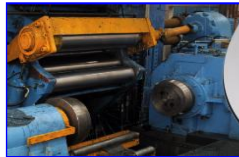
Cold Rolling Mill Coiler
