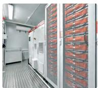
Supply, installation and maintenance of a 75 kW/150 kWh battery storage system for grid-connected and island operation at the JRC-IET.
