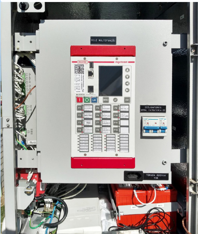
INGEPAC DA PT installed in a cabinet
