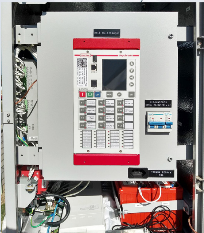
Ingepac DA PT installed in a cabinet
