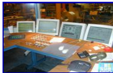
Main Control Pulpit
