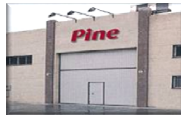
■ CENTRAL WAREHOUSE (VIZCAYA)
