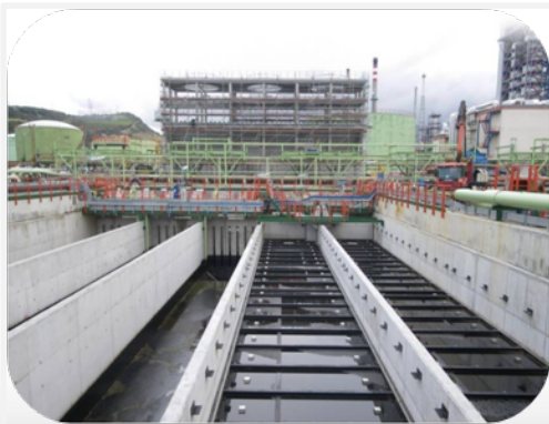
Reinforcement of water treatment in WWTP
