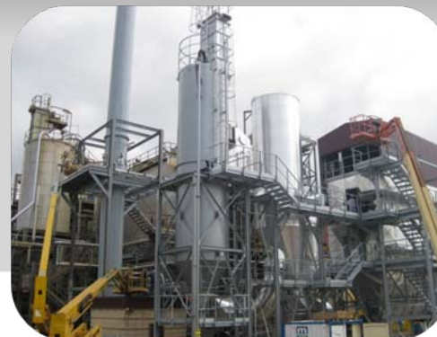
Waste Water Treatment Plant CONSORCIO DE AGUAS
