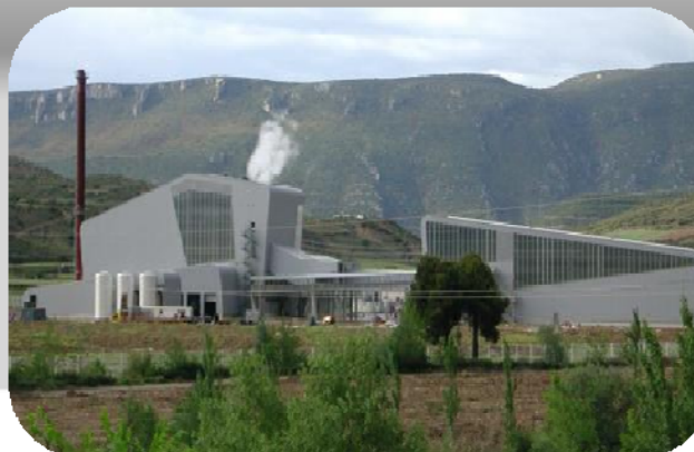
SANGÜESA Biomass Plant
