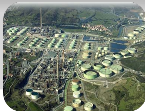
Coke Plant PETRONOR-REPSOL
