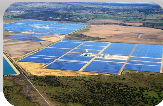
TERMOSOL - Solar-thermal plant
