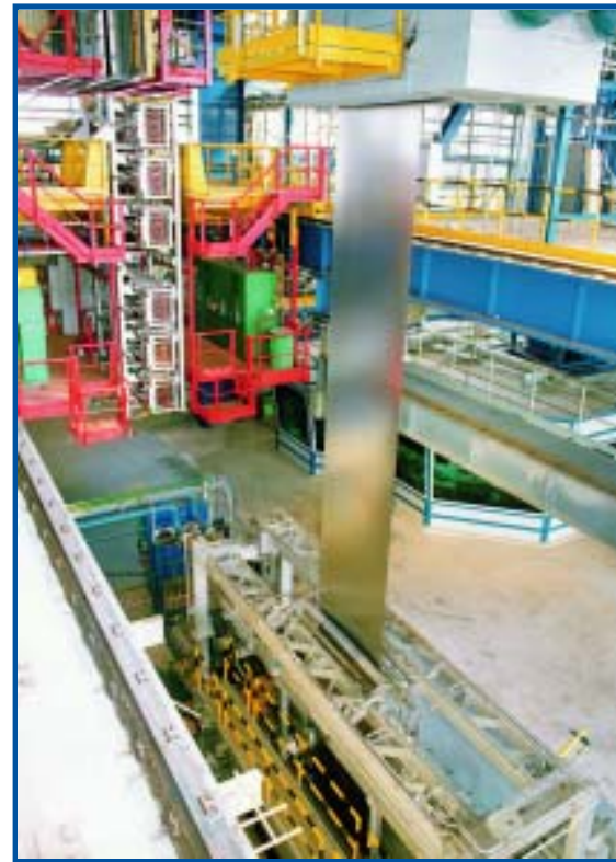
Strip Exit to Cooling Tower
