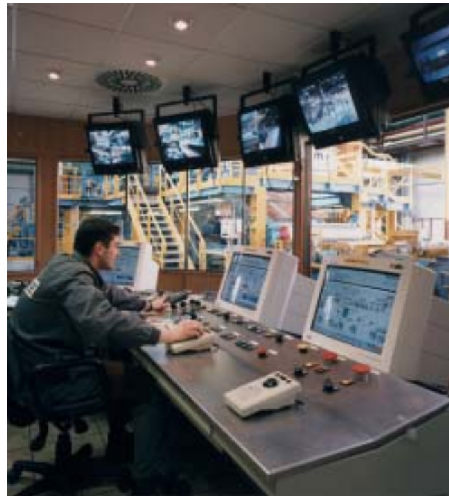
Main Control Pulpit
