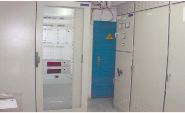
Furnace Regulation Equipment
