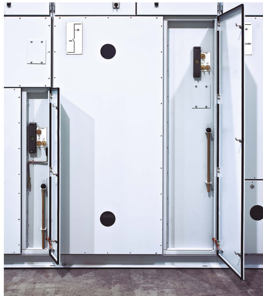
Key interlocking logics by electric equipment key
