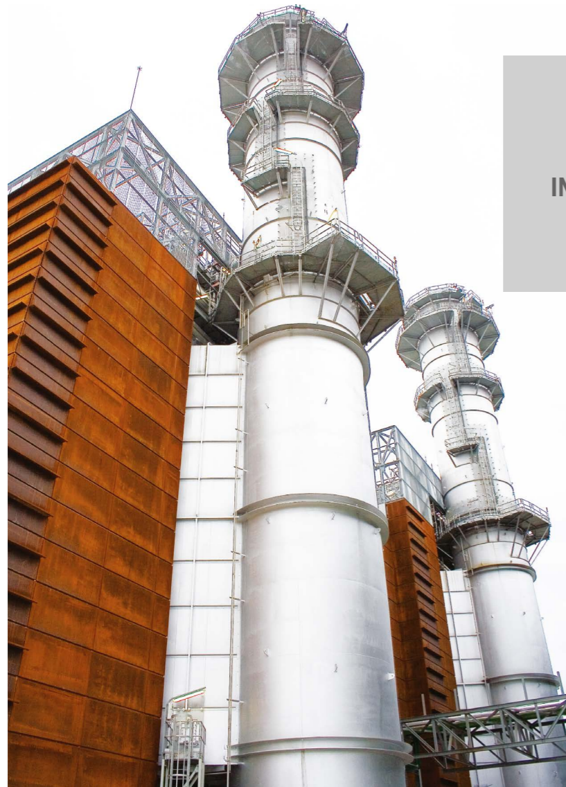
Combined-cycle Power Plant
