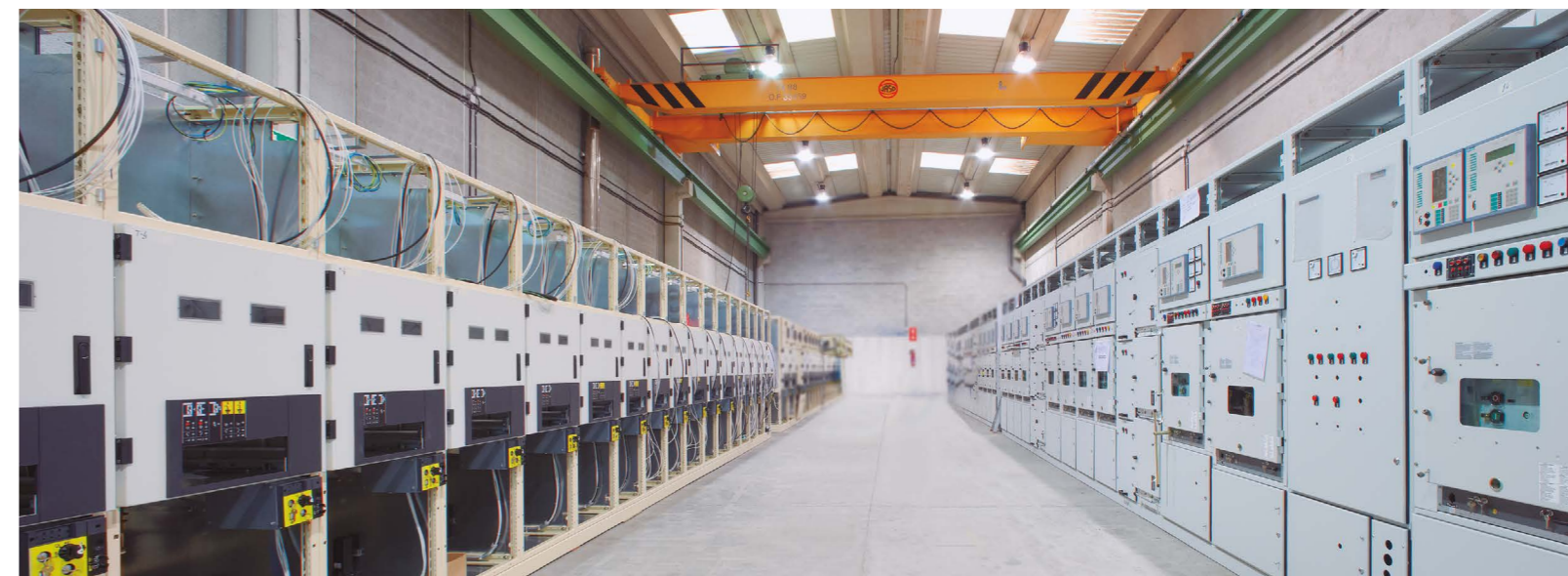
Industrial unit in Pine Zamudio (Spain)
